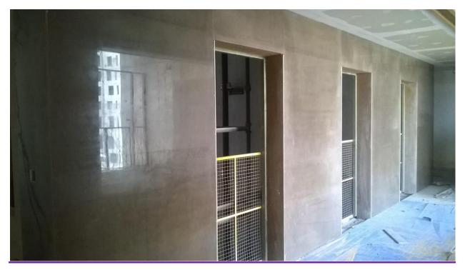
BLOCK WORK COMPLETED. PLASTER & PUTTY, MEP, FLOORING, FALSE CEILING, CARPENTRY WORK IN PROGRESS
